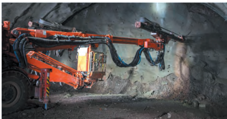
Fig. 7. Drilling of blast holes [3]
