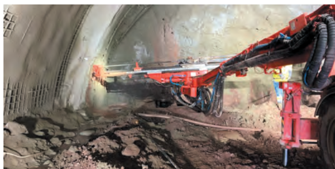
Fig. 9. Execution of primary lining (here: installation of rock anchors) [3]
