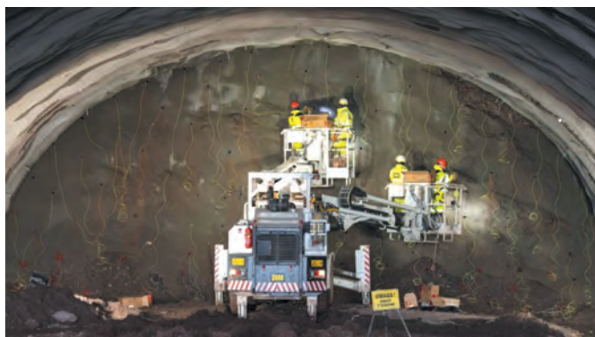
Fig. 8. Setting up explosives [3]
