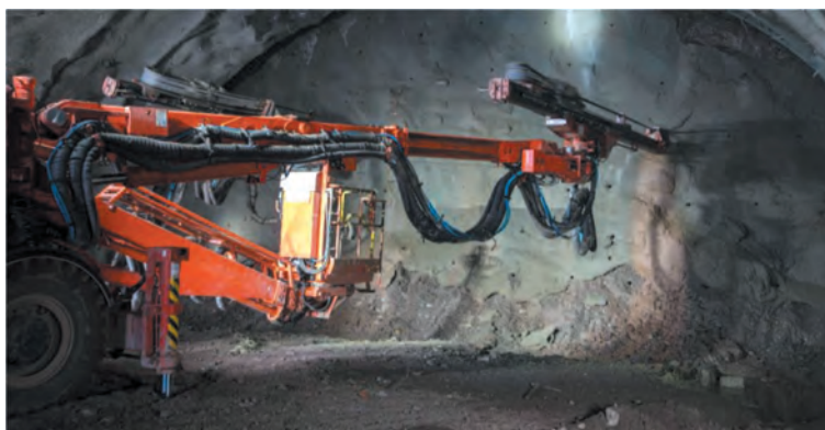
Fig. 7. Drilling of blast holes [3]
