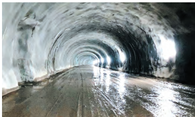
Fig. 12. Tunnel after completion of excavation, completion of the shotcrete levelling layer and technological road [3]
