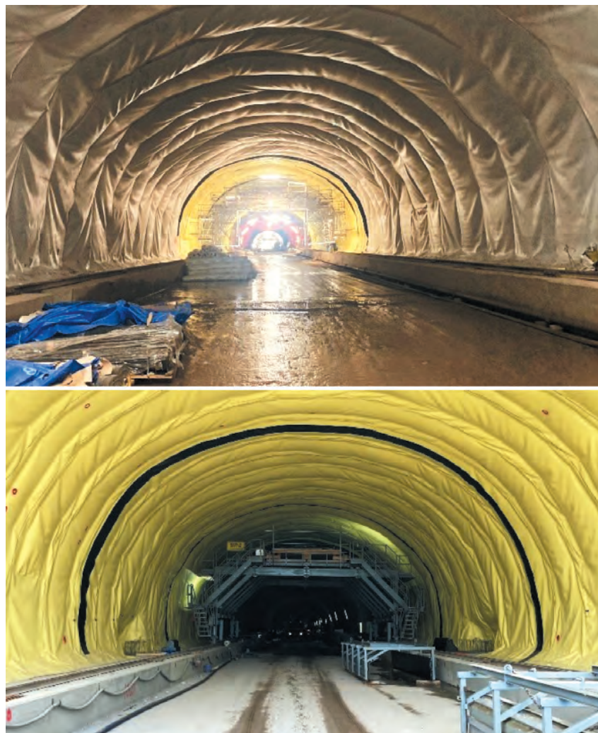
Fig. 13. Execution of waterproofing: geotextile protective layer, PVC membrane [3]
